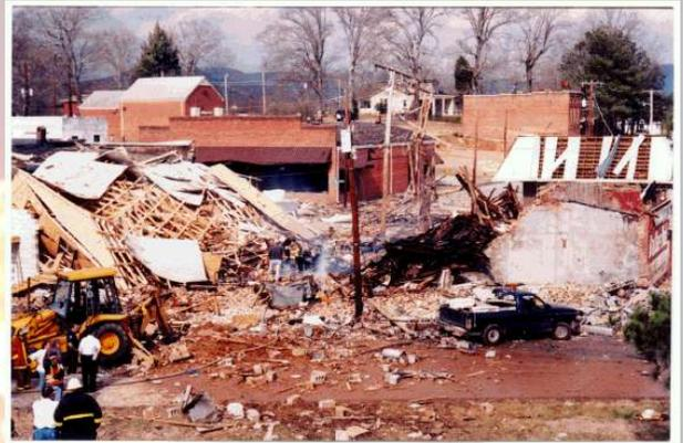
In the pictures above you can see that a backhoe snagged a 3/4" gas line. It was plain to see that the line was damaged at the dig site. What nobody could see was that the gas line was pulled apart underground at the building wall several hundred feet away. While they were repairing the leak at the excavation site, gas seeped into the building and it exploded. **If you expose or damage a gas line while digging, contact a gas representative immediately, or call 911 and report the incident.**
