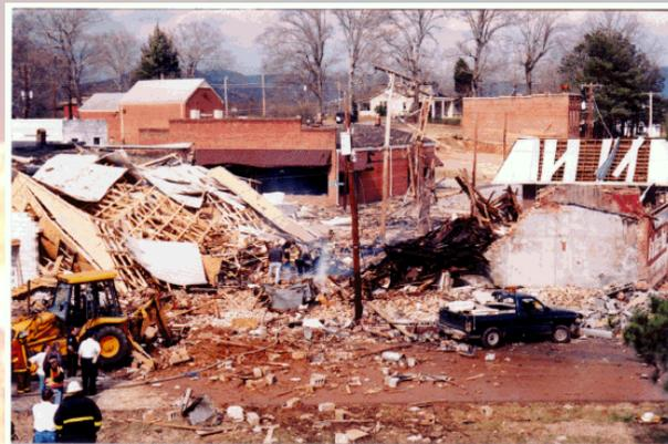
In the pictures above you can see that a backhoe snagged a 3/4" gas line. It was plain to see that the line was damaged at the dig site. What nobody could see was that the gas line was pulled apart underground at the building wall several hundred feet away. While they were repairing the leak at the excavation site, gas seeped into the building and it exploded. **If you expose or damage a gas line while digging, contact a gas representative immediately, or call 911 and report the incident.**
